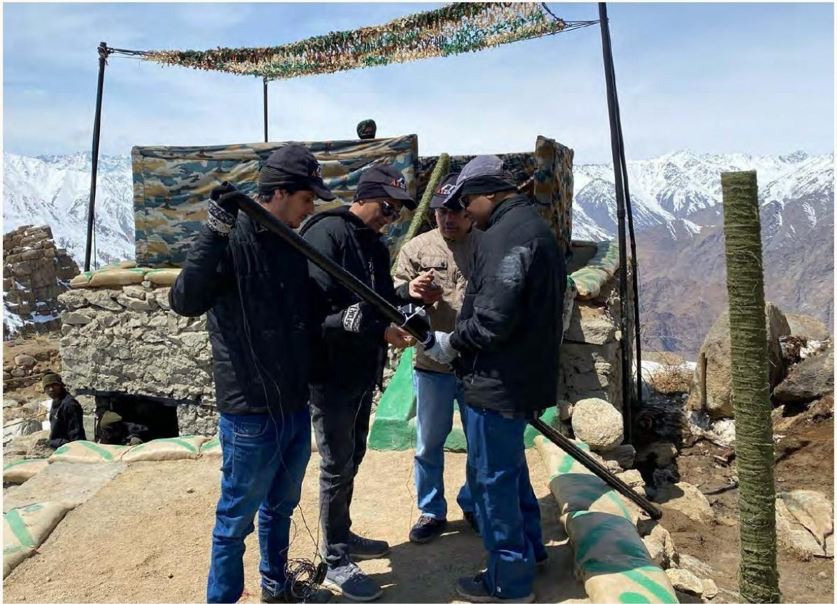
Mounting End-fed 10-40M antenna with Spiderbeam mast
